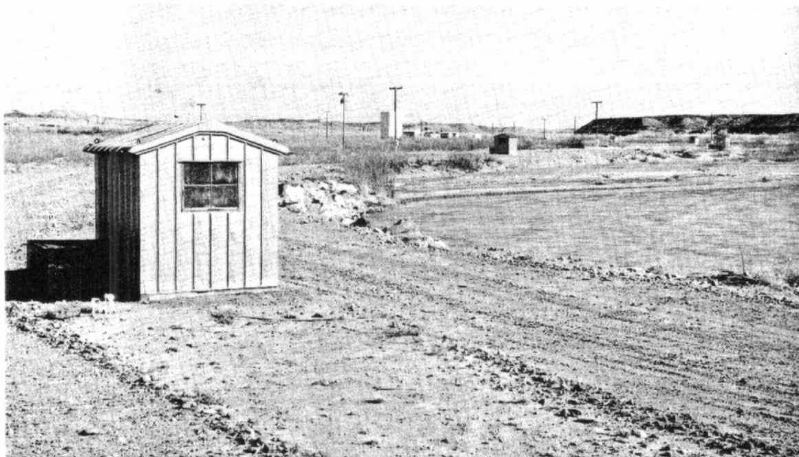
Pumps on wells driven into the gravels along the banks of the San Juan River. The well water is pumped into oil structures at the nearby Aneth field to increase oil recovery.
