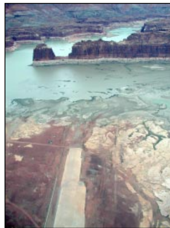
Hite Marina boat ramp, decommissioned by sediment
