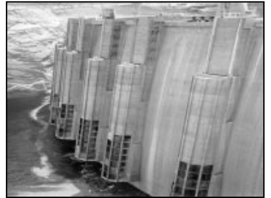
Glen Canyon Dam intake towers to be modified
